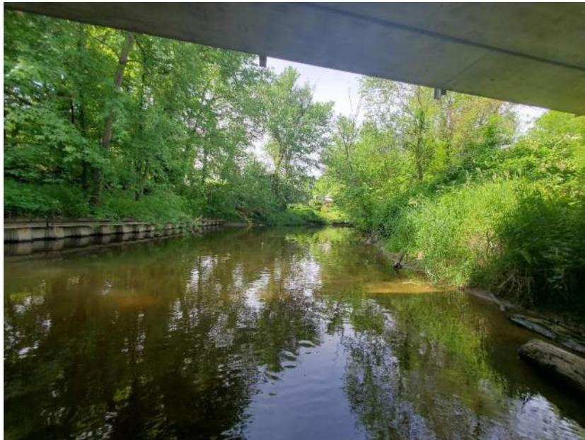
Photo 7. View under CR 26 Bridge, looking south, upstream of Baugo Creek, showing bank conditions. Note the steel sheet piling along east bank.
